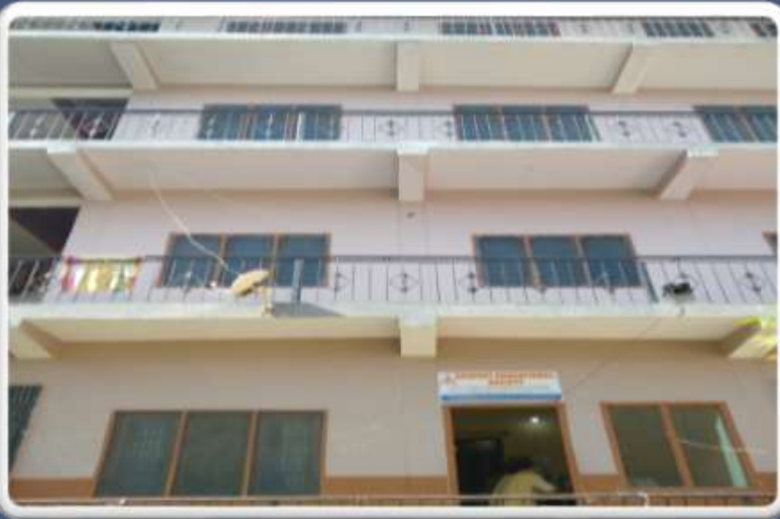
PIC. NO.1 showing building structure of organisation in kunihar .
